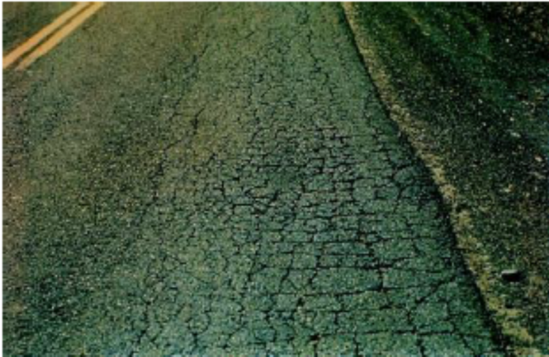
Fatigue Cracking
