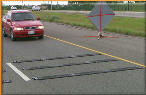
Temporary Rumble Strips
